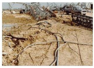
FIGURE 1: CRUMPED STRUCTURE AND GUY WIRES OF THE COLLAPSED TOWER
